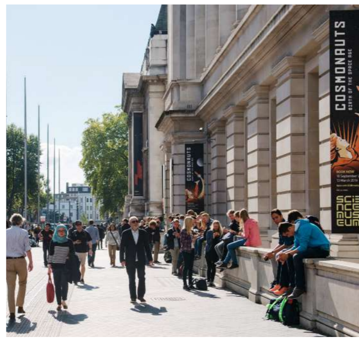
View towards site from Exhibition Road
