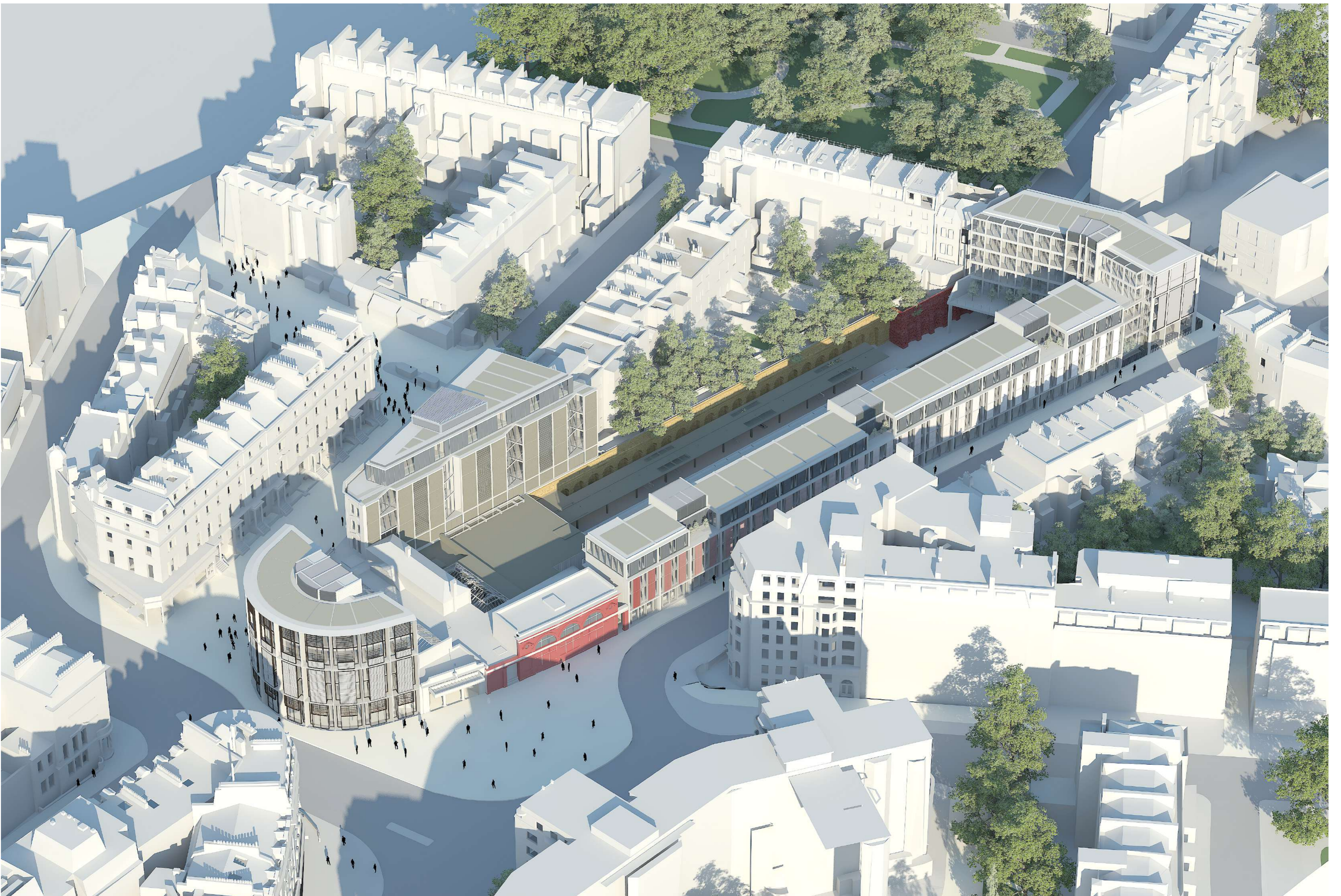
South Aerial View
