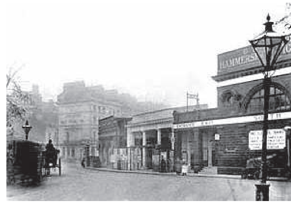
The George Sherrin-designed arcade under construction circa 1907
