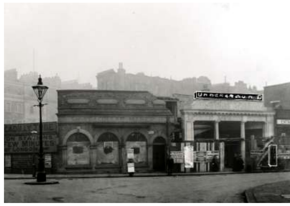
The George Sherrin-designed arcade under construction circa 1907
