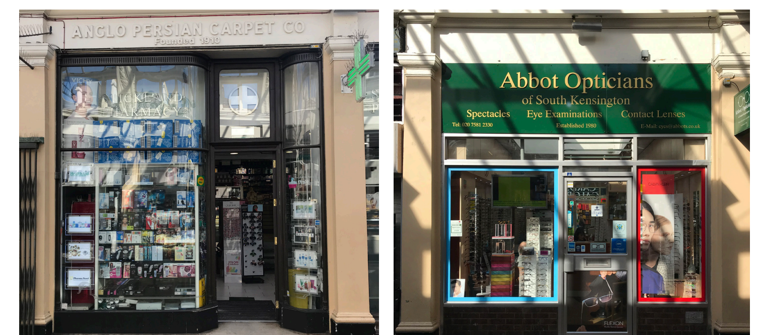
No. 6 - The only surviving original shopfront No. 13 - Non-original shopfront
