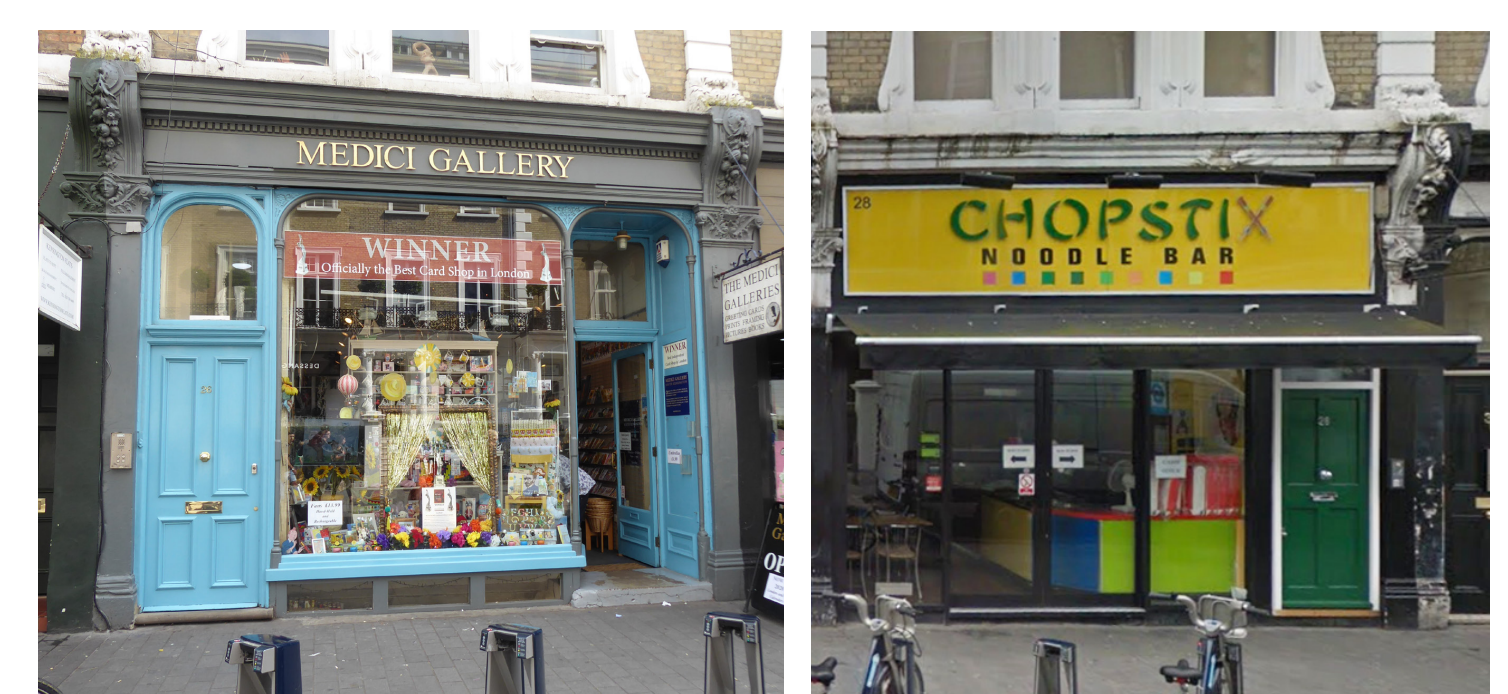
No. 26 - The only surviving original shopfront No. 28 - Non-original shopfront
