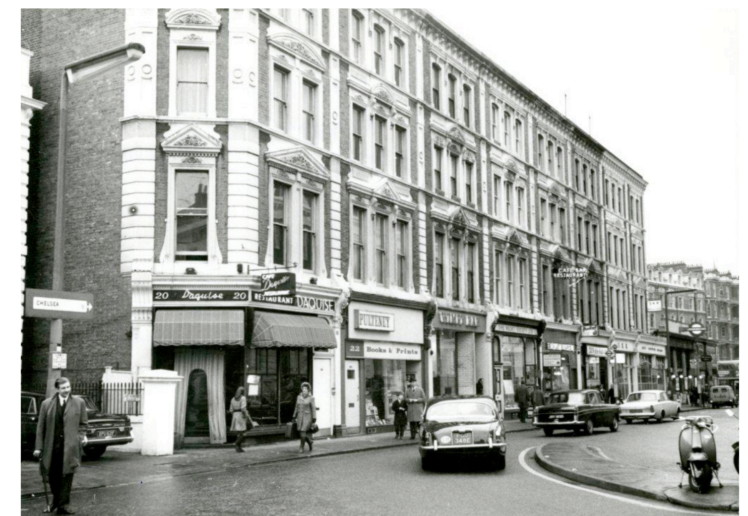
View looking down Thurloe Street c.1970 showing unsympathetic shopfronts
