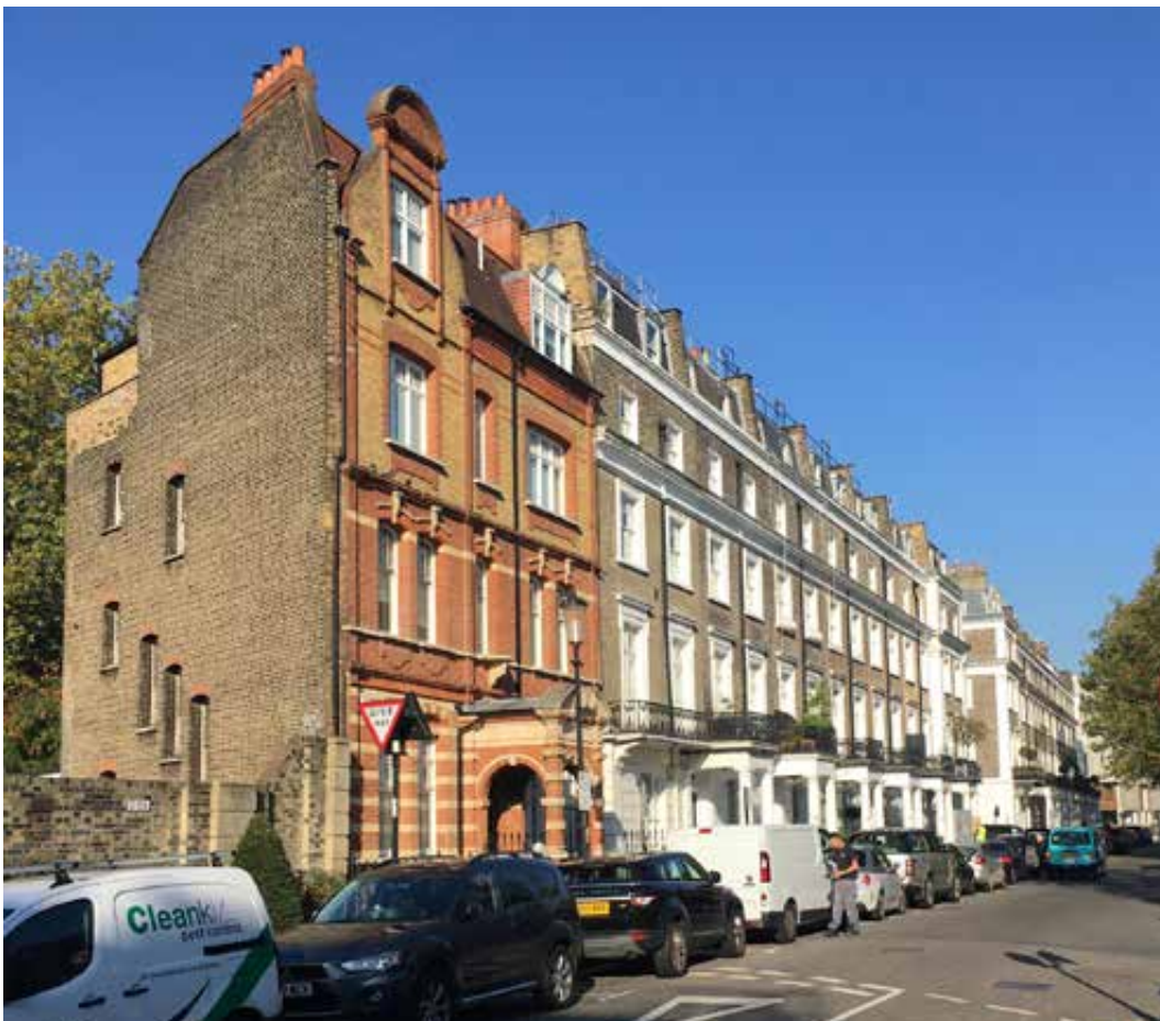
Fig. 16: The western terrace of Thurloe Square with No. 52 Thurloe Square in the foreground
