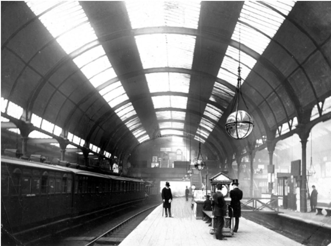
Fig. 41: The southern train shed, c.1900 - Note the cast iron columns which survive today
