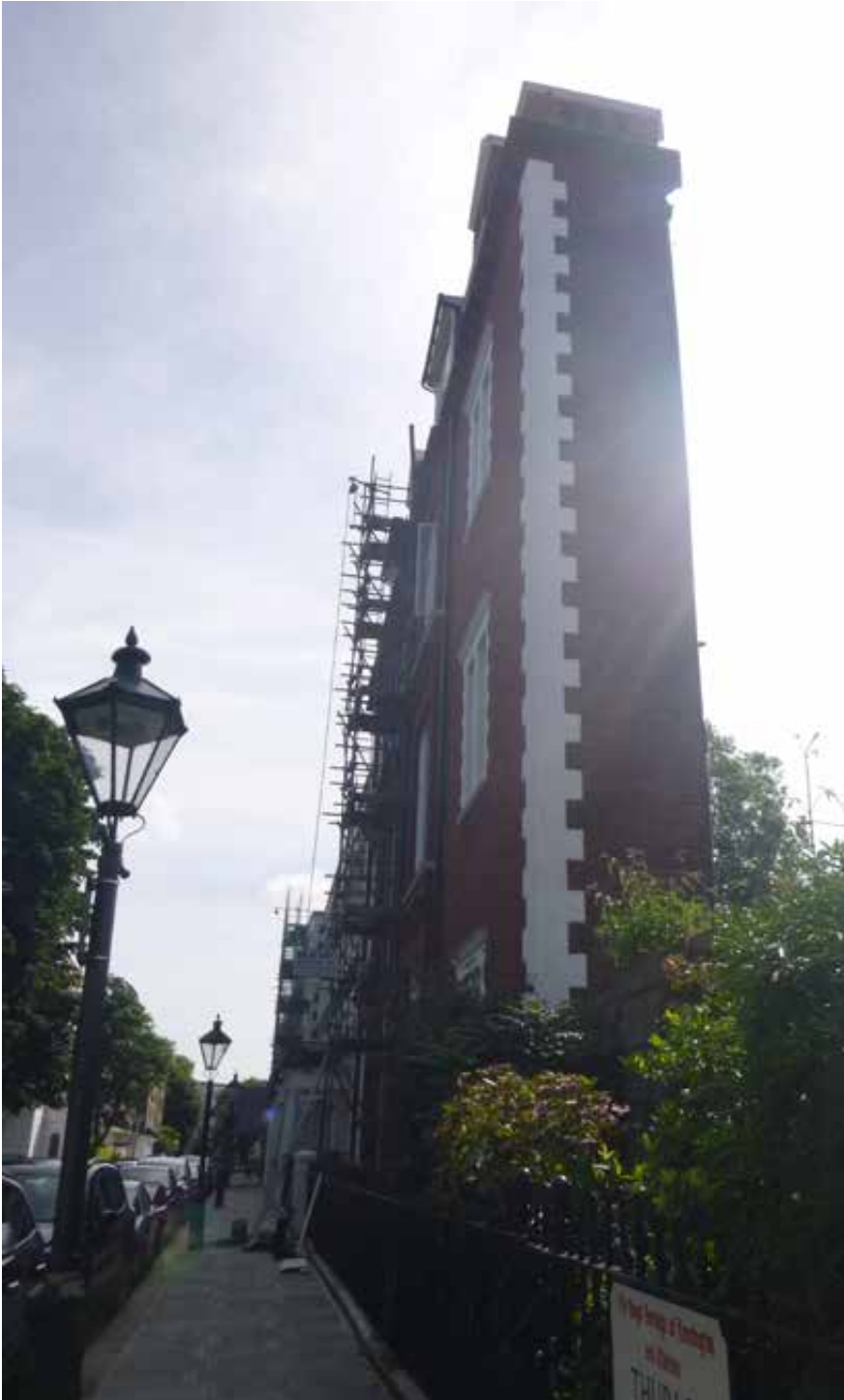
Fig. 18: No. 5 Thurloe Square 'The Thin House'
