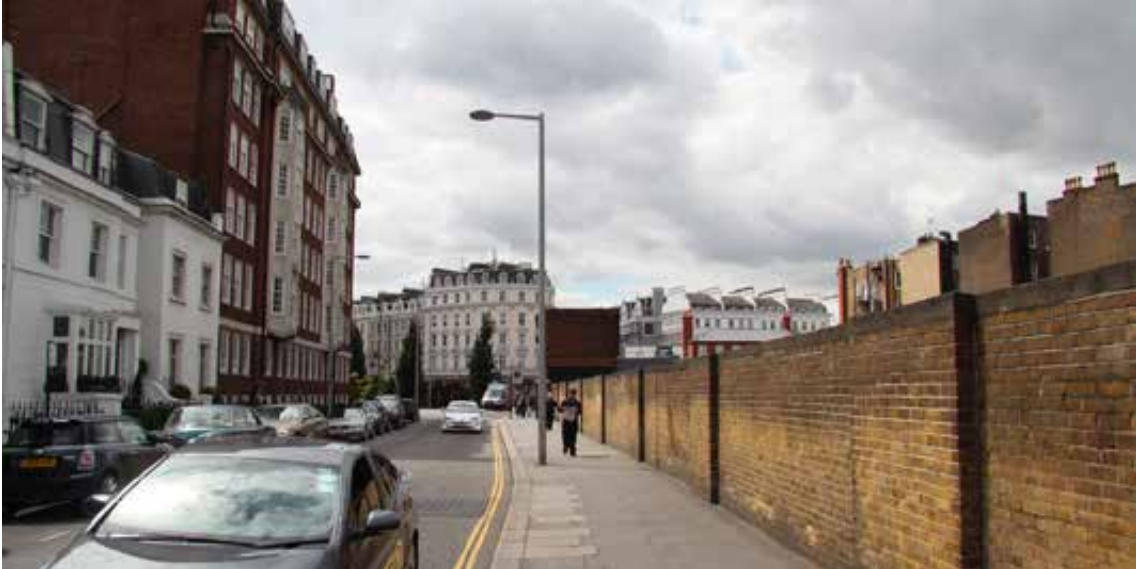
Fig. 14: The wall on the north-side of Pelham Street
